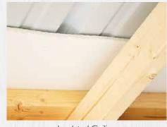
Insulated Ceiling Standard on metal roof option
